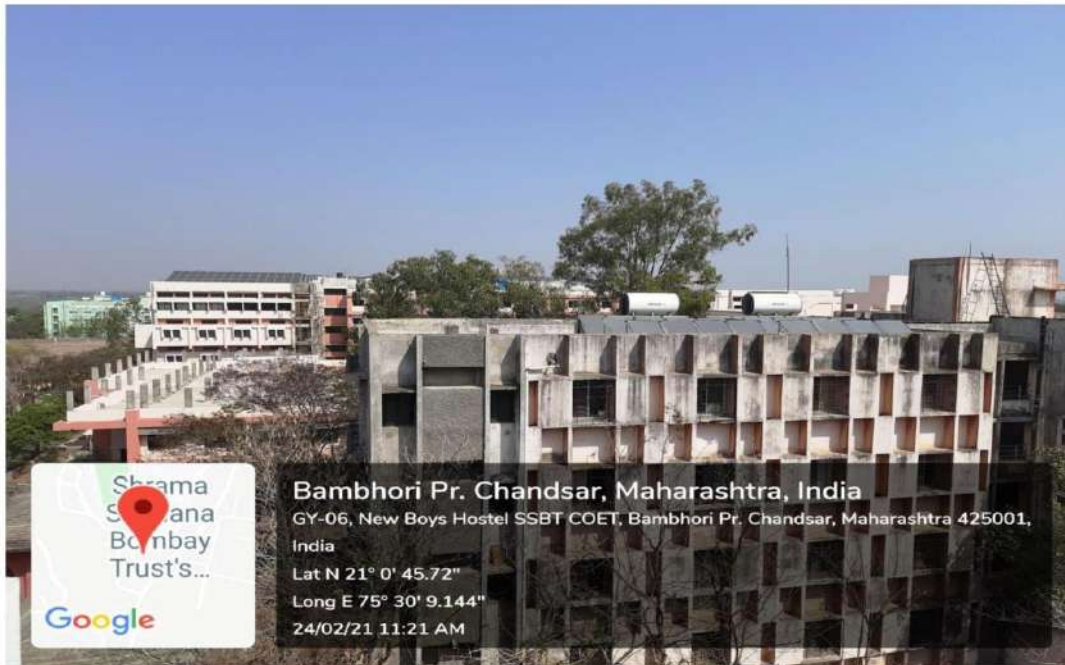
Fig . No. 1 Solar Water Heater at Hostels' Rooftop
