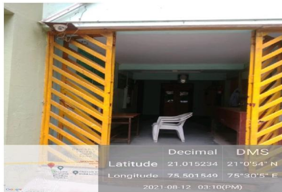
CCTV AT Girls Hostel
