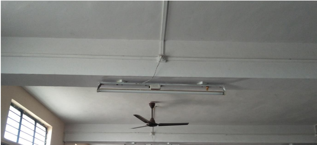
Fig. No.3 Fluorescent Tub Light before Replacement
