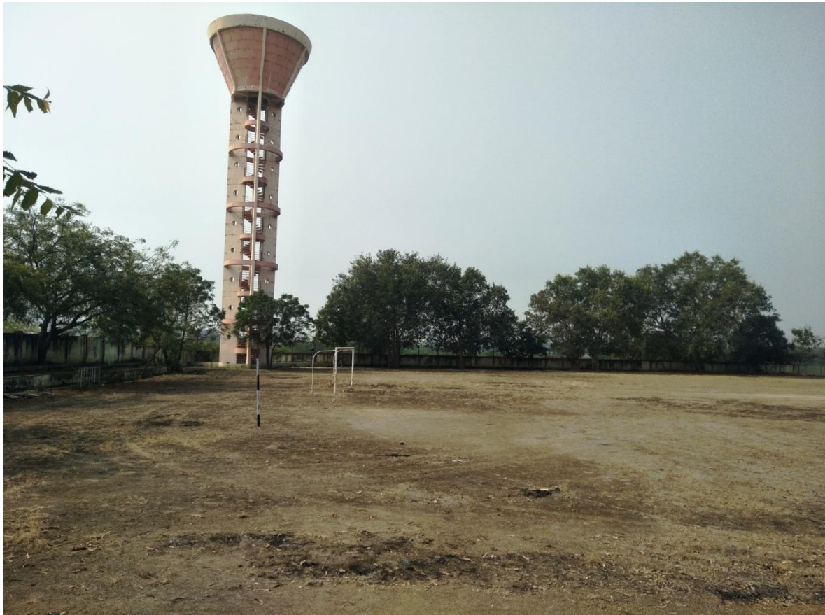
Fig. No. 7 Single over head water tank
