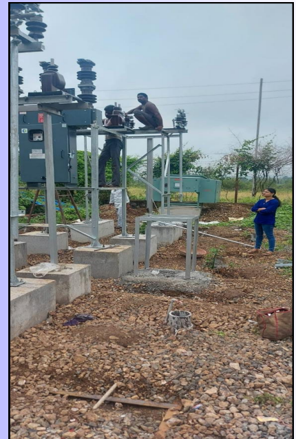
Execution of work at substation
