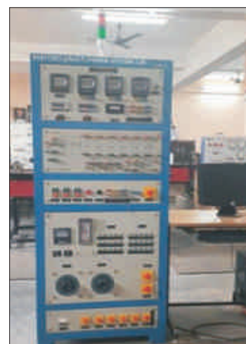
400 KM long Transmission Line
